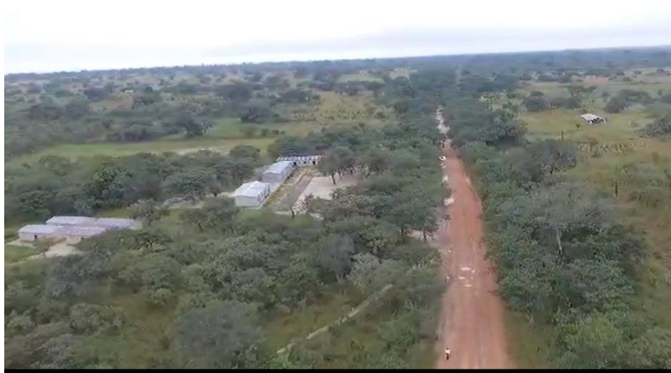
Figure 3: Aerial view of the trunk road for rehabilitation
